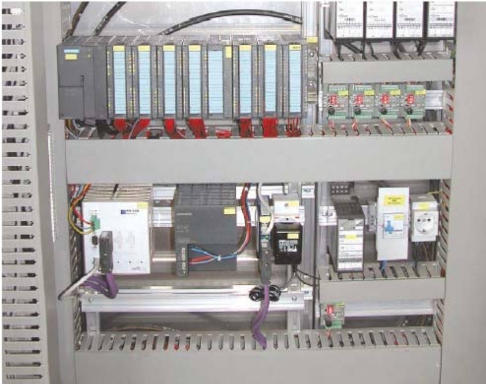
Figur 2: The FG-300 from Softing integrates Profibus and Ethernet via easily accessed interfaces to form a logical network.
