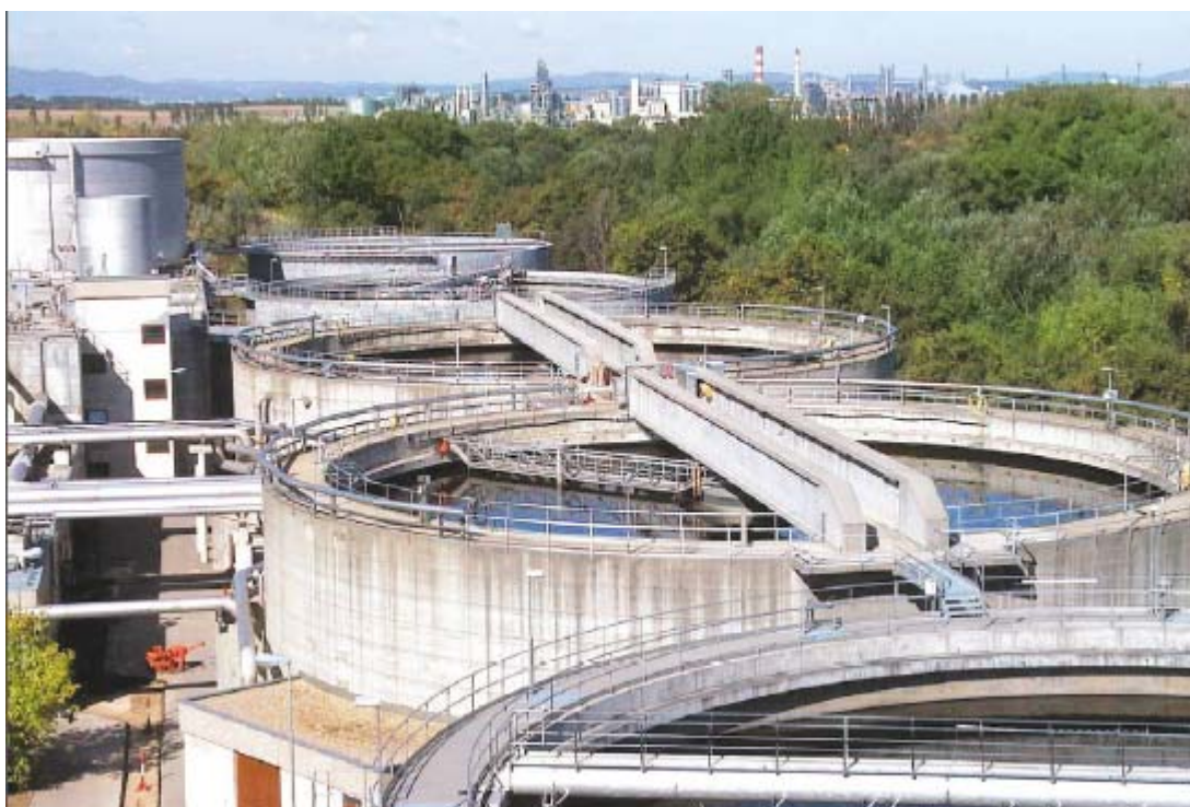
Figur 1: The Schwechat Mannswörth wastewater treatment plant in Lower Austria was established in 1988, modernized in 1995 and most recently equipped with modern Ethernet-Profibus gateways early this year. The field devices can now be configured directly over the data network.
